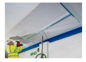
The fixing of plasterboards to ceiling can cause manual handling injuries caused by the strain of lifting plasterboard above their head. Using a panel lifter supports the plasterboard allowing one person to fix the plasterboard with better posture and reducing the strain on their body.
